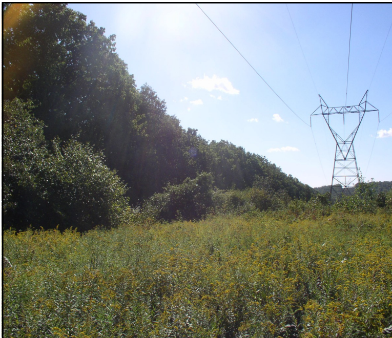
Herbaceous critical wire zone at mid-span, surrounded by shrubs in the adjacent wire zone and border zone.
